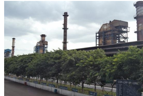
Power Plant: 12 MW & 2.5 MW
